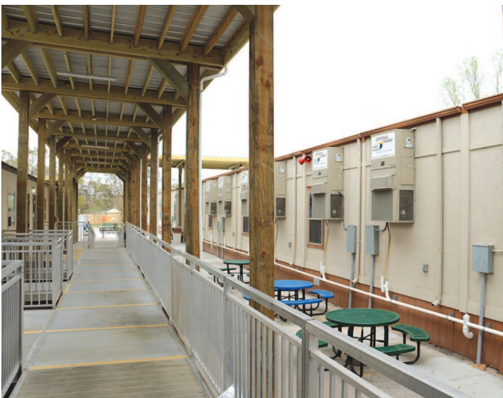
The temporary campus for St. Margaret of Scotland Catholic School includes 25 individual modular buildings strategically placed together and connected by approximately 2,500 square feet of elevated walkways and covered awnings.
