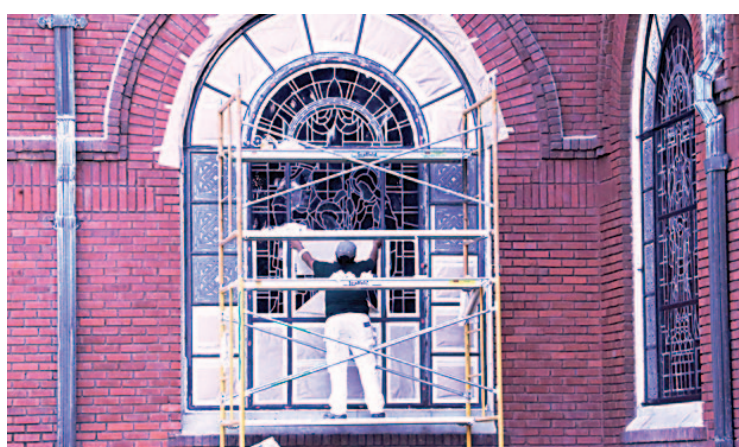
Using scaffolding a worker blocks stained glass on windows
