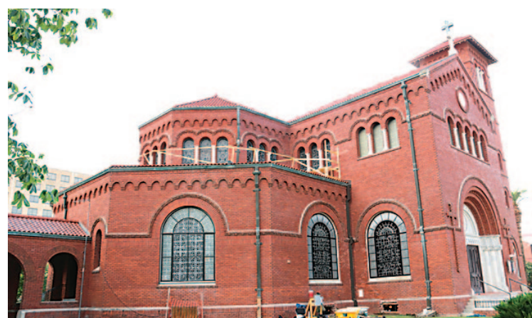
Scaffolding in place on upper windows of Cathedral
