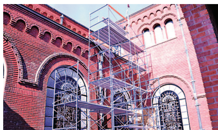
North courtyard scaffolding allows access roof
