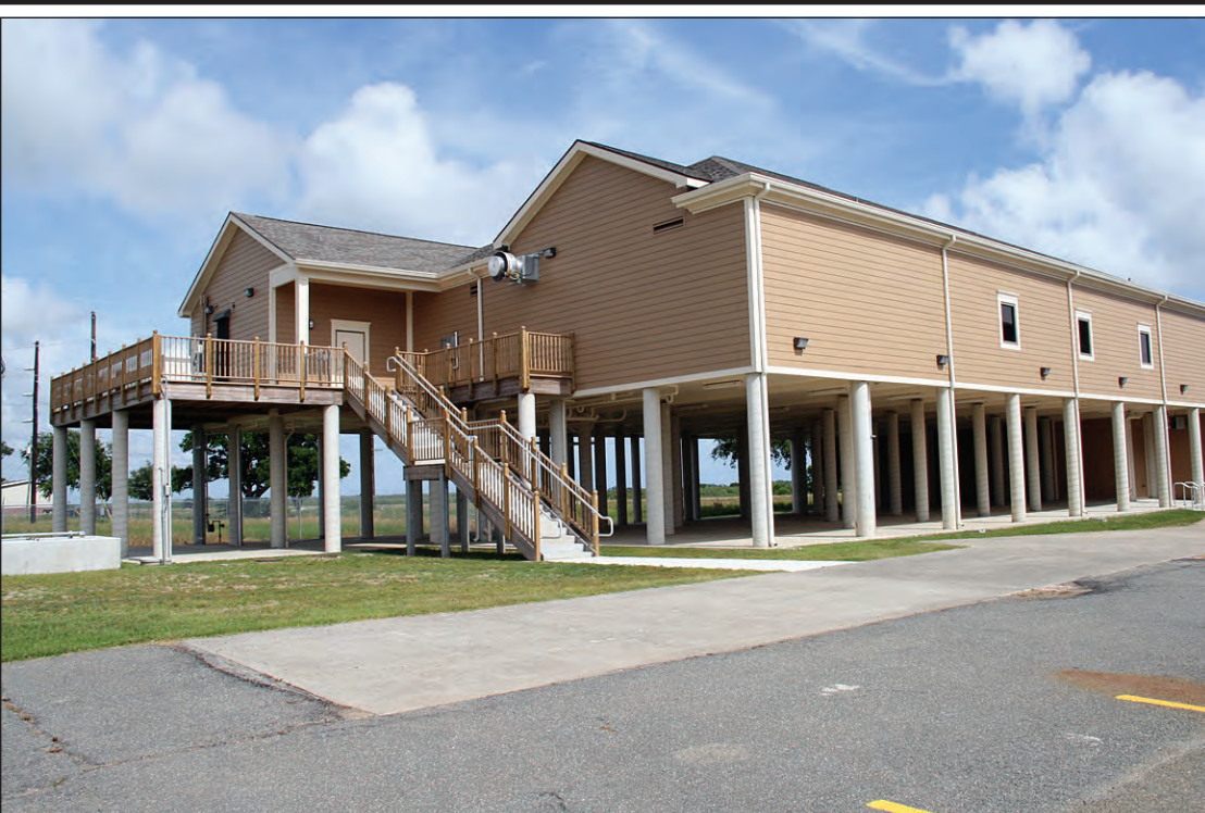
The newly completed Sacred Heart of Jesus / Our Lady Star of the Sea Life Center is shown in the left photo. The building is 142 feet by 72 feet in size with 7,790 total square feet perched 19 feet six inches above sea level. There are 12 rooms, including five classrooms, two offices, a 3,118 square feet multipurpose room, kitchen and restrooms. It is of raised wood frame construction on reinforced concrete pilings and concrete col-
