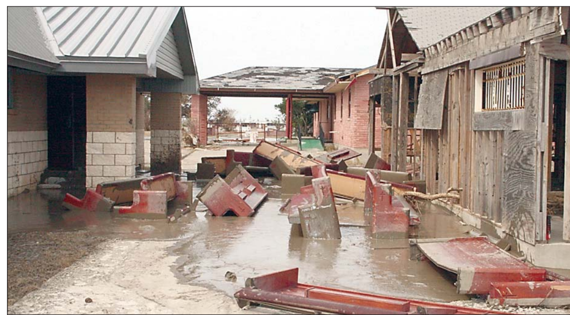
Pews deposited outside of Sacred Heart Church
