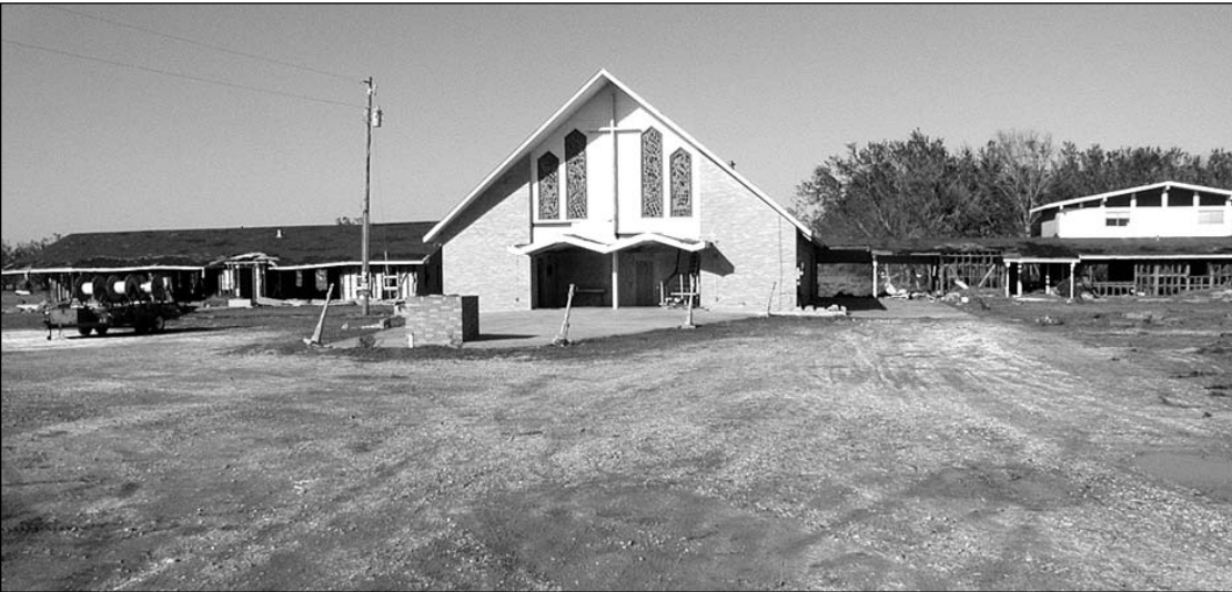
Like most structures in Cameron Parish lying as close to the Gulf of Mexico as St. Eugene does, the storm surge pounded the church, hall and rectory leaving devastation in its wake.
