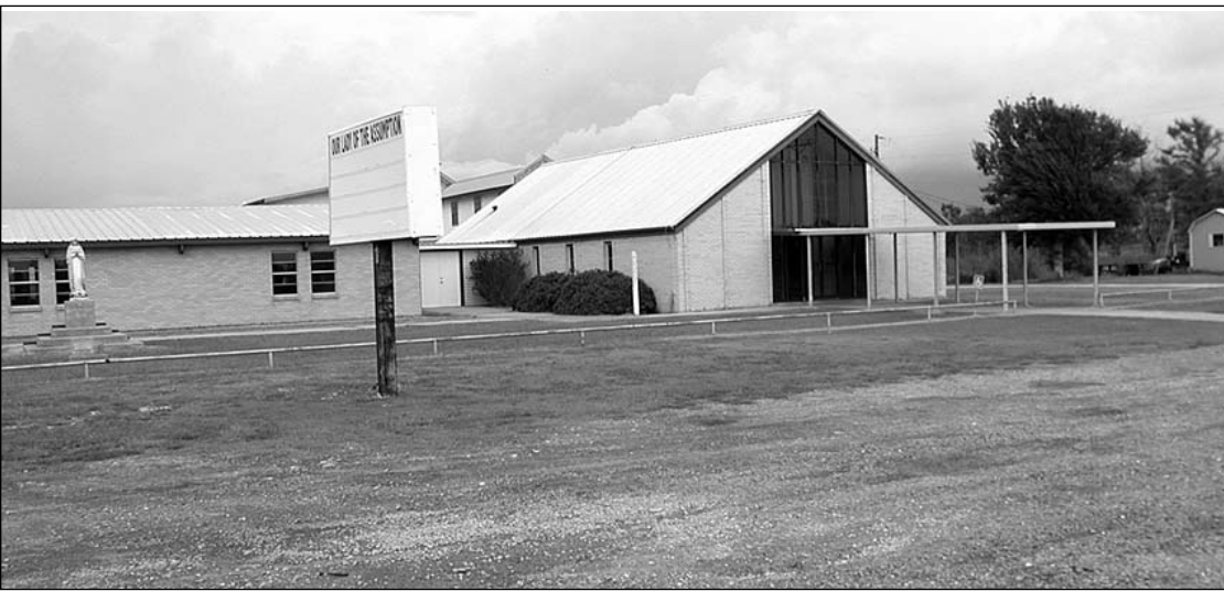
The Chapel of the Assumption in Johnson Bayou, the closest church building to the point of landfall of Hurricane Rita, and its rectory and religious education building have been repaired and Liturgy has been celebrated there since Sunday, April 16 - Easter Sunday.
